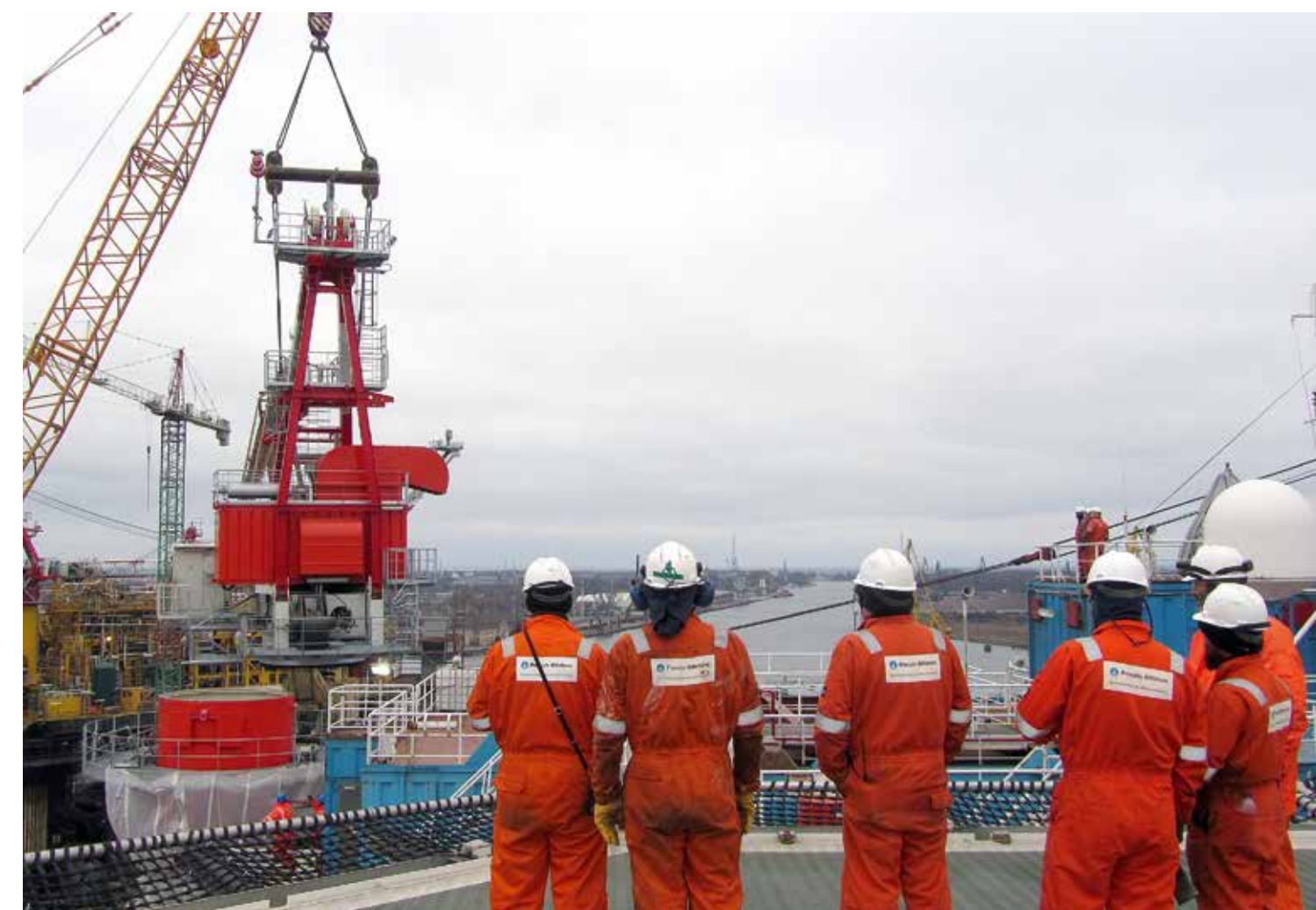
Installation of the Liebherr deck crane 17 metres high and weighing 70 tons on-board the Safe Bristolia . The crane was lifted up 44 metres in the air and then precisely lowered onto the rig's deck.
